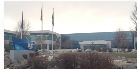
Source: Governor's Office of Energy
