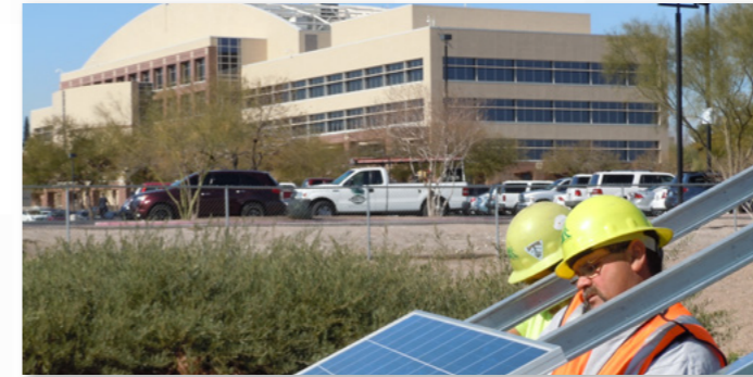
Grant Sawyer Building, Las Vegas
