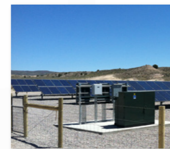
Source: Lincoln County Power District No. 1
